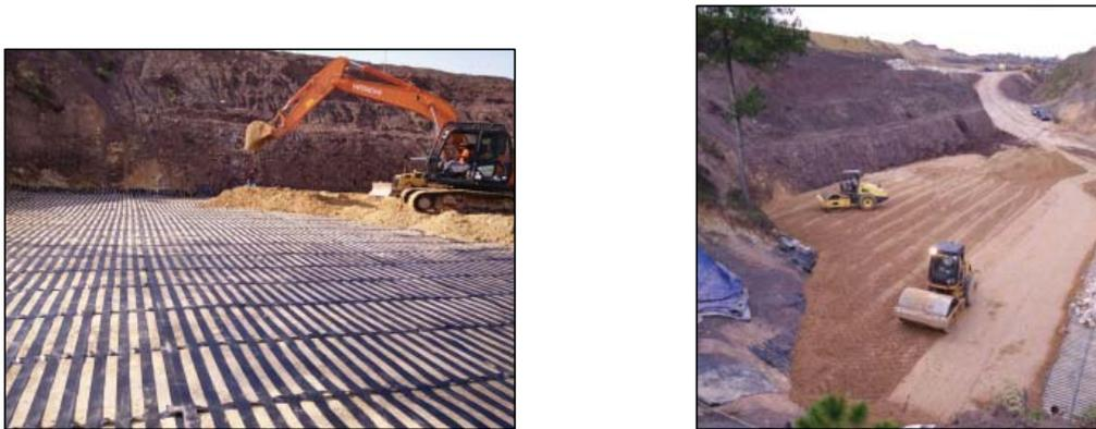
**Fig. 11:** Tana Toraja RSS under construction (backfilling and compaction operations)
